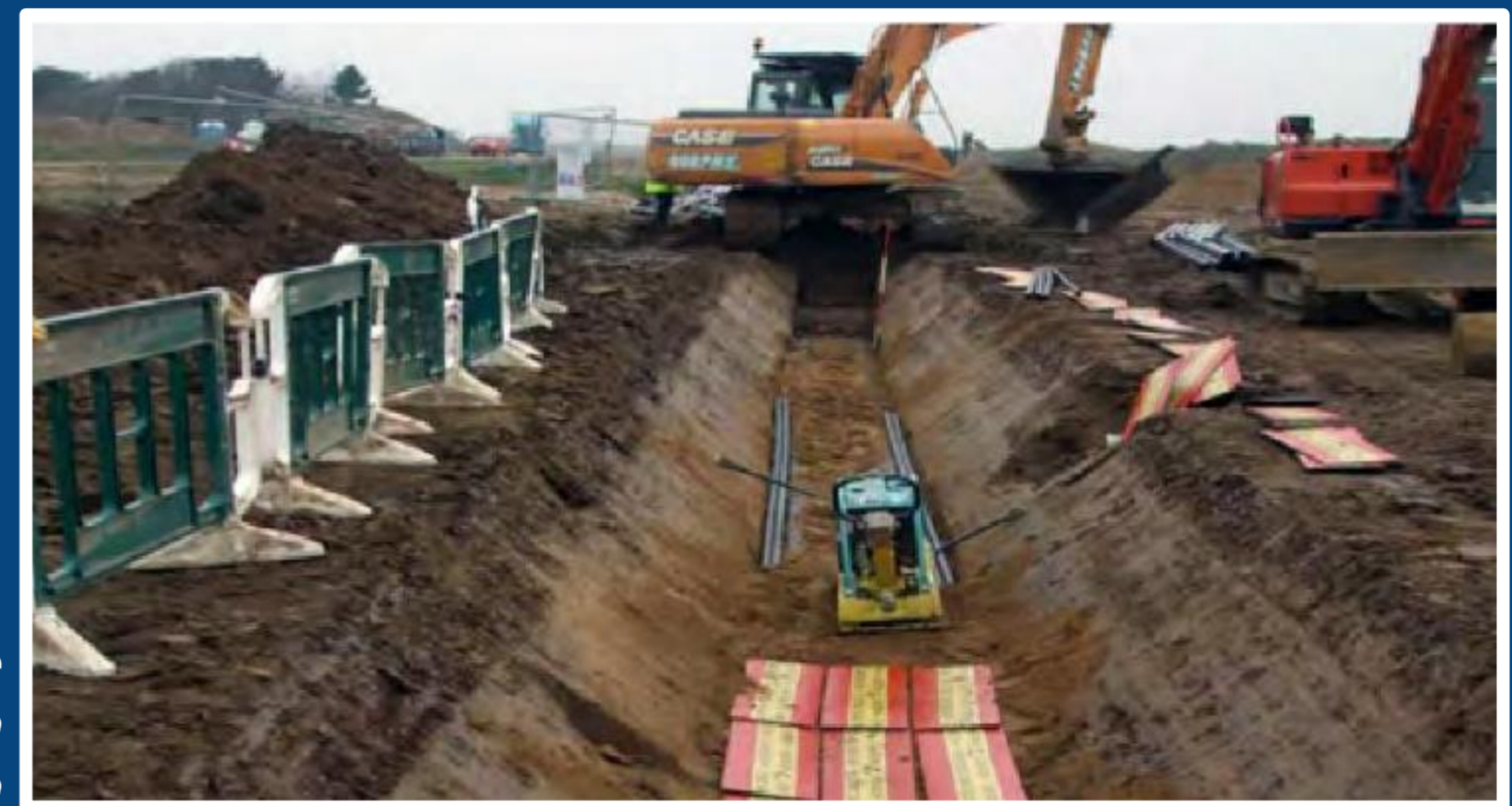
Typical cable installation operation
