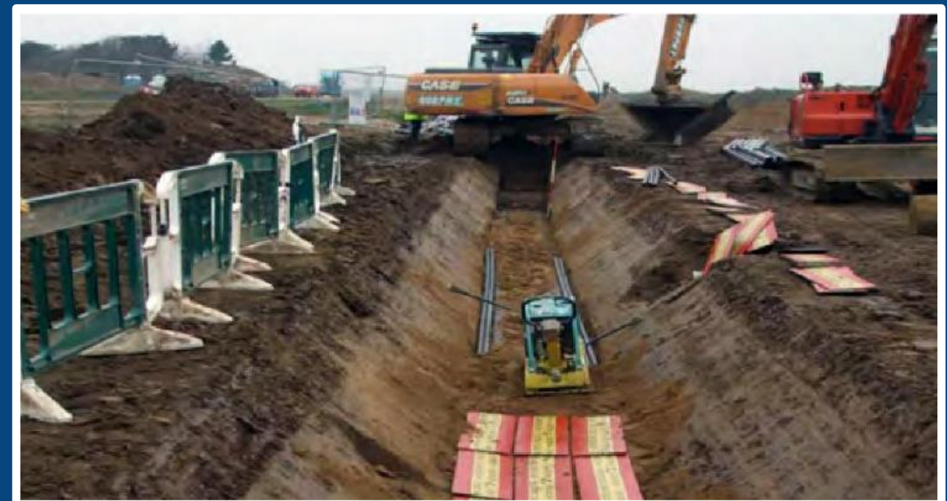
Typical cable installation operation
