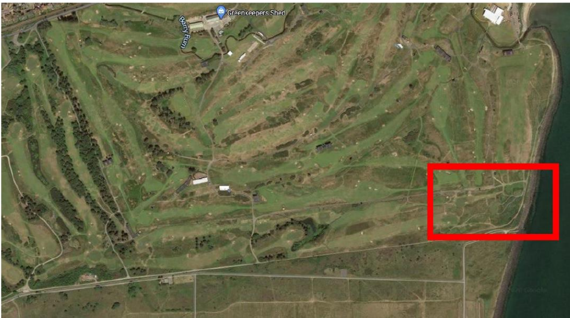
Fig 2 – Landfall works area located at Carnoustie Barry Golf Links.
