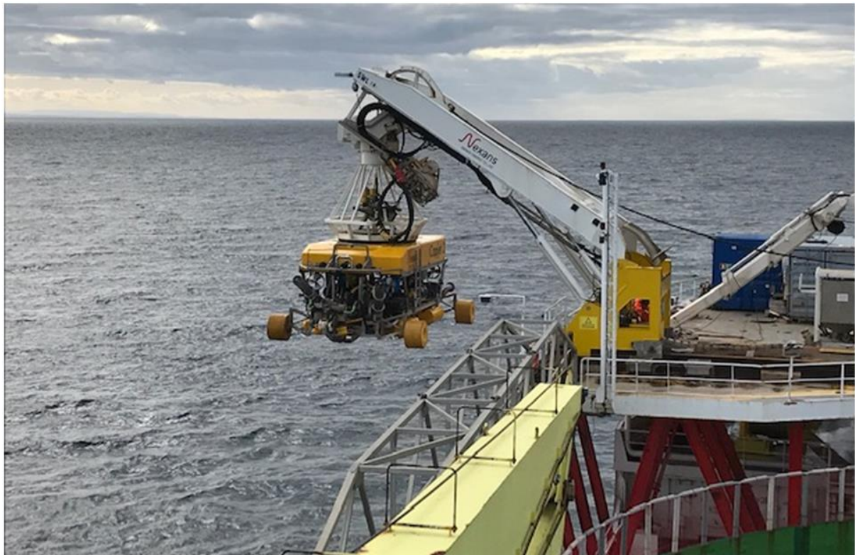
Fig 3 – Capjet trenching tool deployment.
